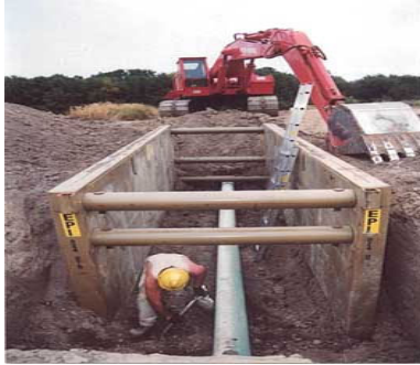
Trench box during water line installation
