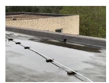
Water ponding on roof near drain
